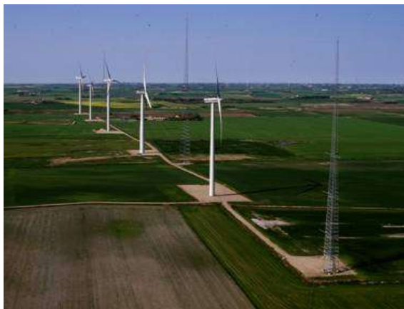
Figure 2: Høvsøre test site, showing MW class turbines and met. masts on test stands
